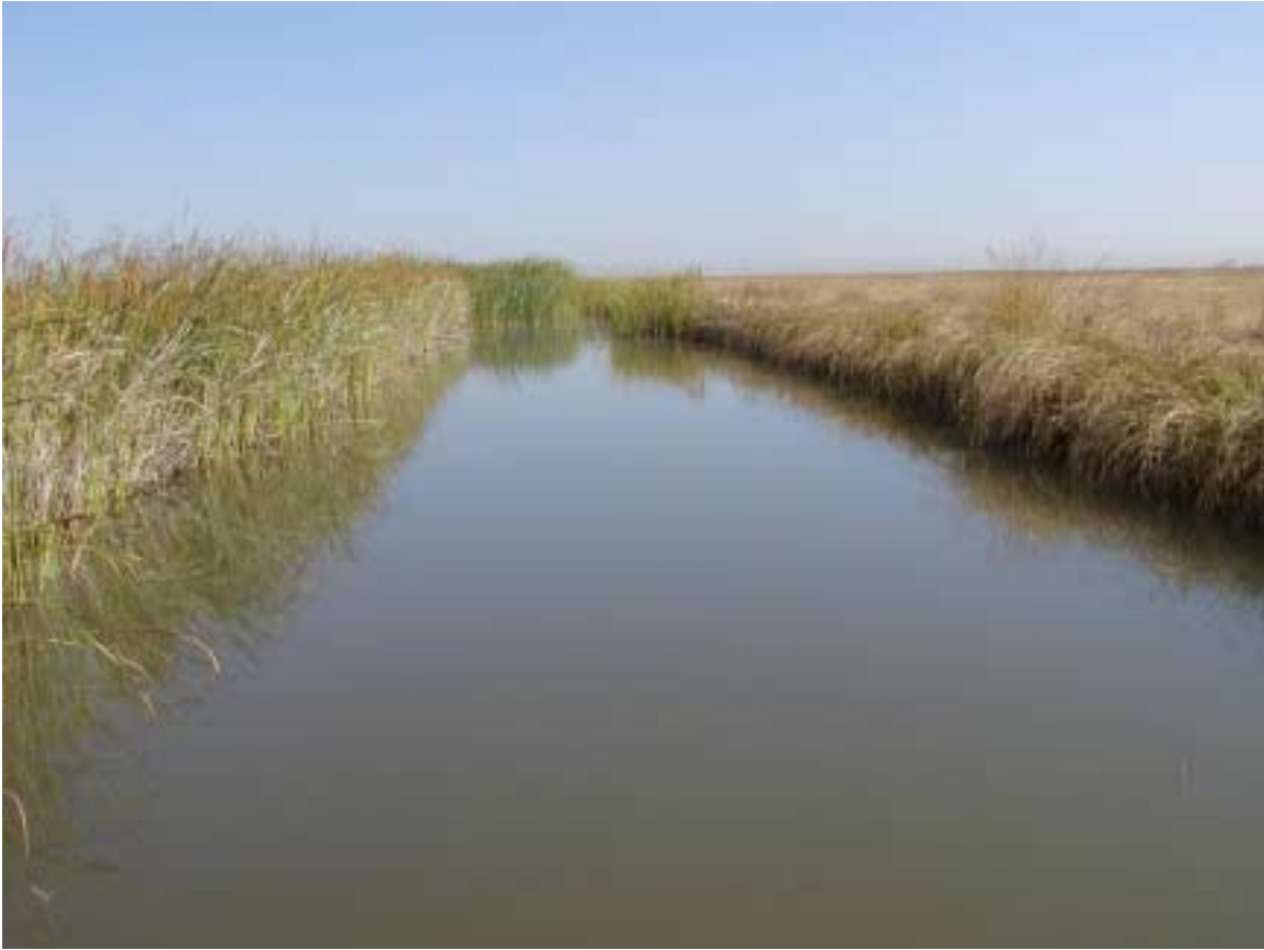
Ditch off of Elkhorn Road.
