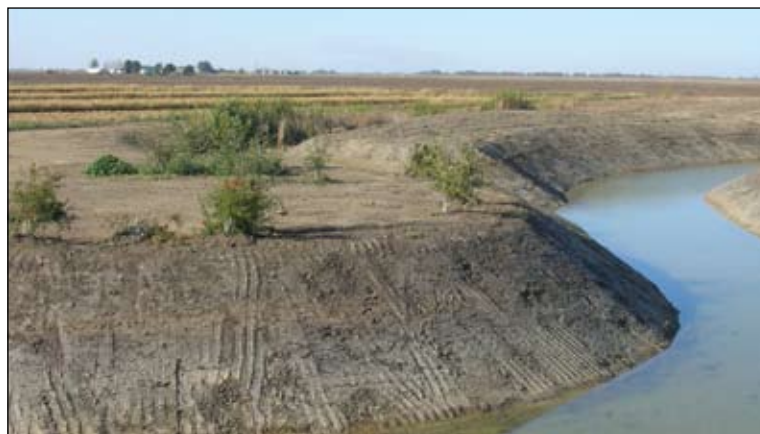
Figure 1. Channel clearing and maintenance results. On the Lucich South managed marsh complex, channel clearing efforts have been completed. The photo at right shows a restored channel prior to full flood-up. Note earlier-planted native shrubs and trees preserved in channel clearing process.
